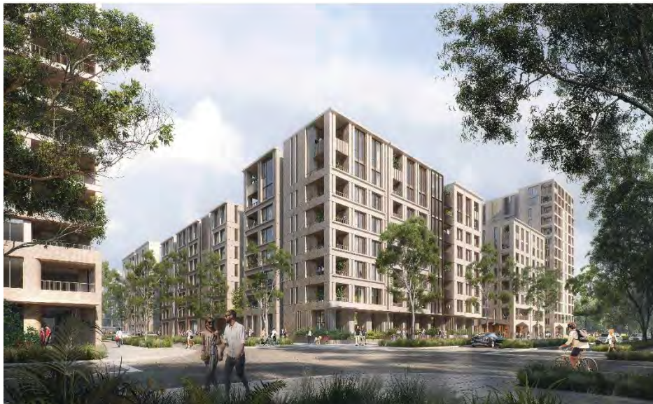
Figure 2: View from North East, corner of Zetland and Defries Avenue
